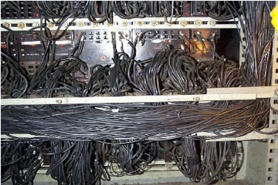
100G wire occupies less than half of the volume of the wire used in this installation
